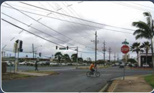
Frontage road running parallel to Farrington Highway
